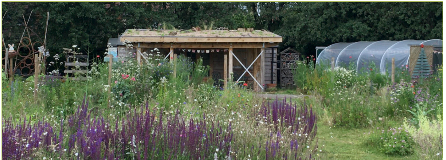
24 June 2021: The day we installed the green roof on the veranda.
